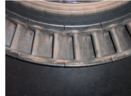
Fouling on HPT stator blades, [2]
